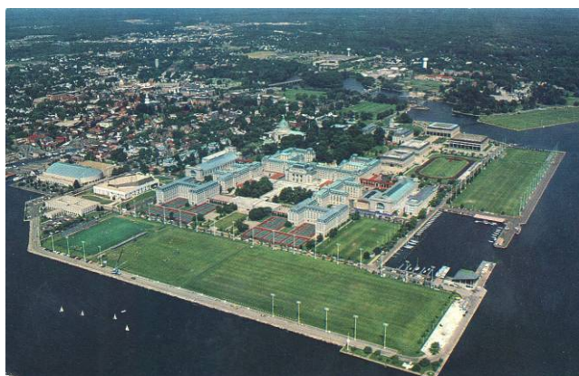
Aerial View of the Naval Academy at Annapolis
